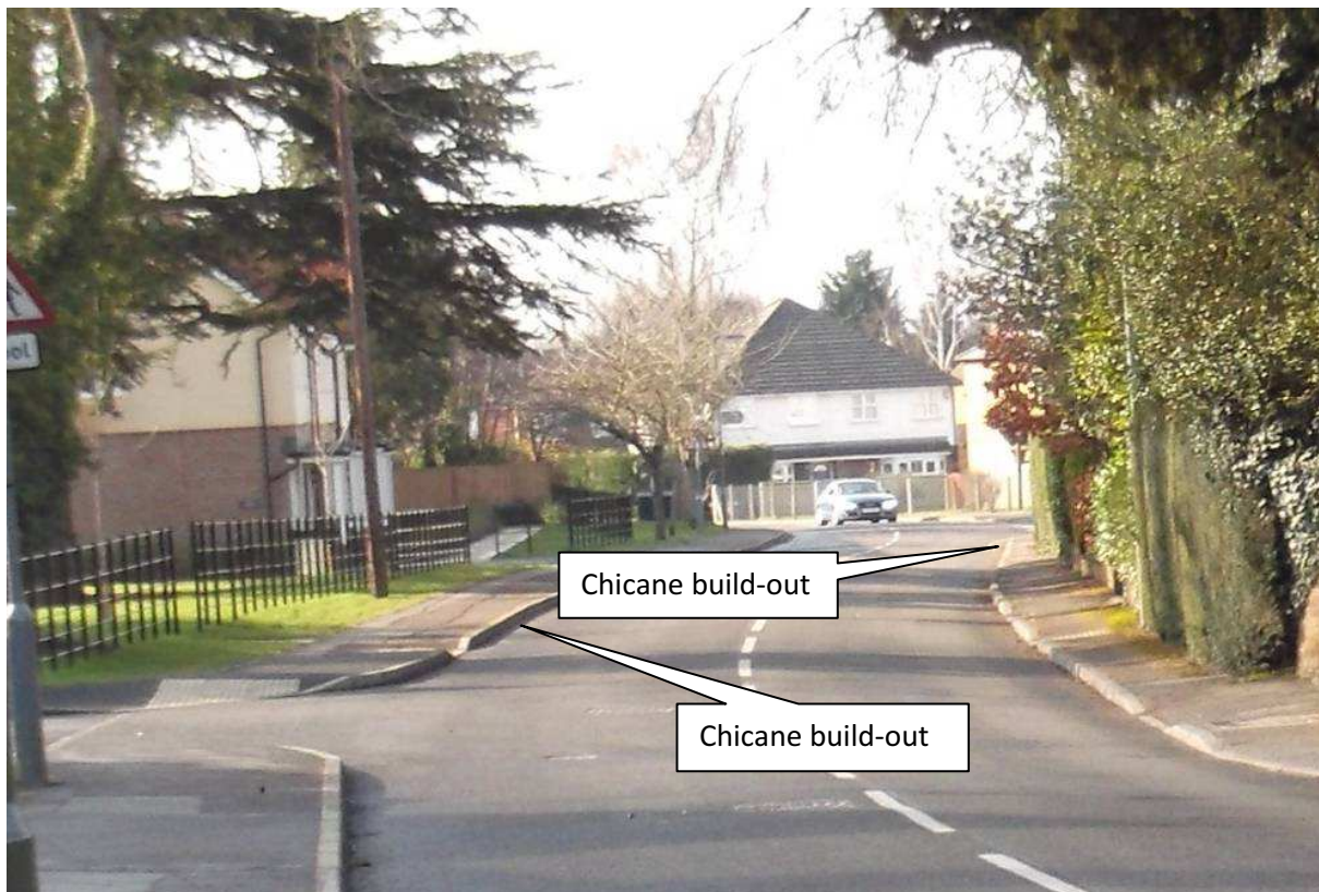
Existing crossing point near the junction with Mulberry Way
